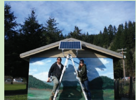
Alsea Community Effort, Alsea Emergency Power System
